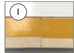
I. When inserting the last two screws, take care to not let the ends separate and create a gap.
